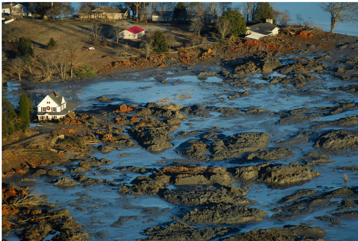
A dike on a coal ash pond ruptured at the Kingston Fossil Plant in Tennessee, in December 2008, spilling 1.1 billion gallons of toxic sludge across 300 acres. It damaged or destroyed 40 nearby homes, polluted the Emory and Clinch Rivers with coal ash, and cost $3 billion in clean up and economic impacts. PHOTO: Dot Griffith via Appalachian Voices.
