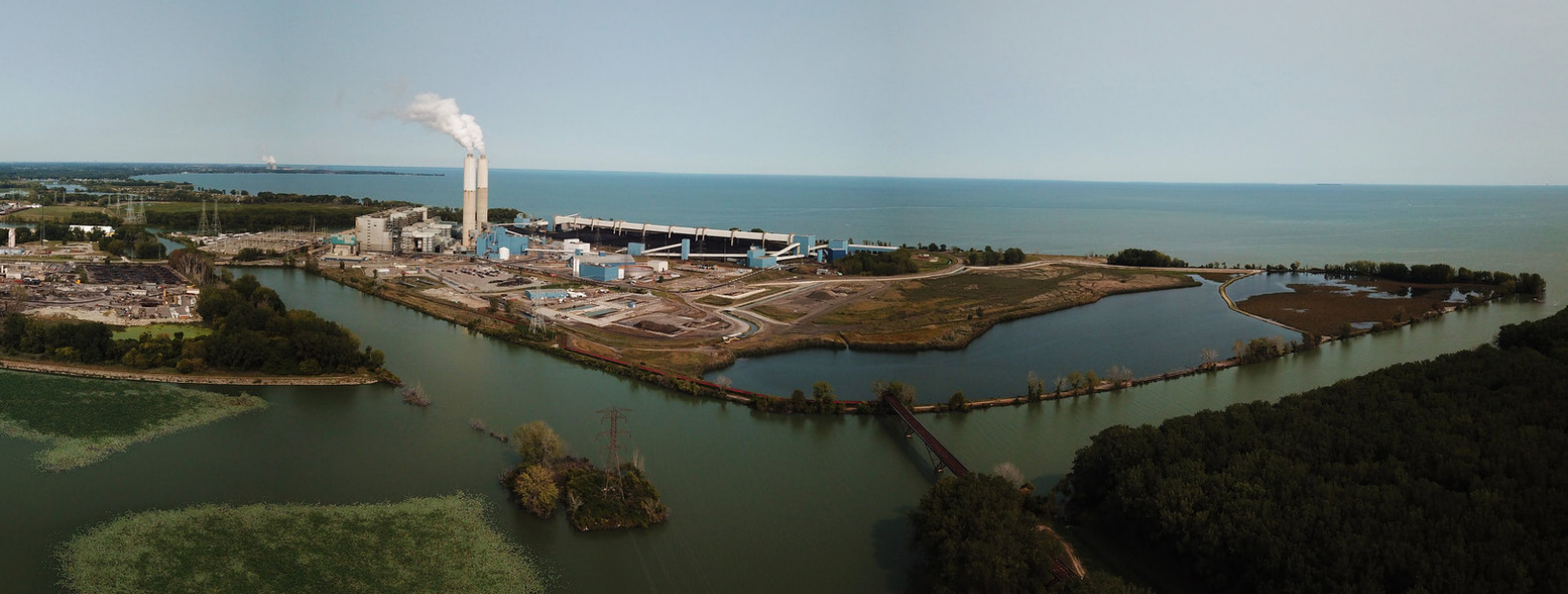
DTE's Monroe bottom ash pond was constructed in Lake Erie by taking a low area of the lake and building up an earthen dyke to separate the holding pond from the lake. PHOTO: Ted Auch, FracTracker Alliance, 2020.
